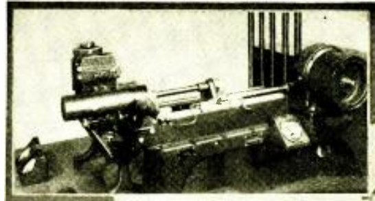
Right Photograph of the transmitter. The motor may be seen at the left and the amplifier and oscillator at the extreme right.
